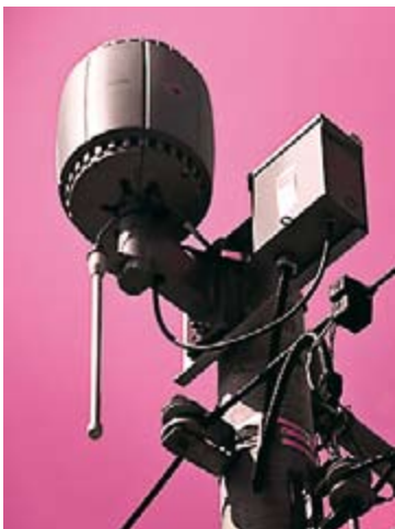
Information technology: one of the "kegs" used by Toronto Hydro in Canada to provide WiFi to city-dwellers across 235 city blocks. © Flickr Creative Commons/Marc Lostracco
